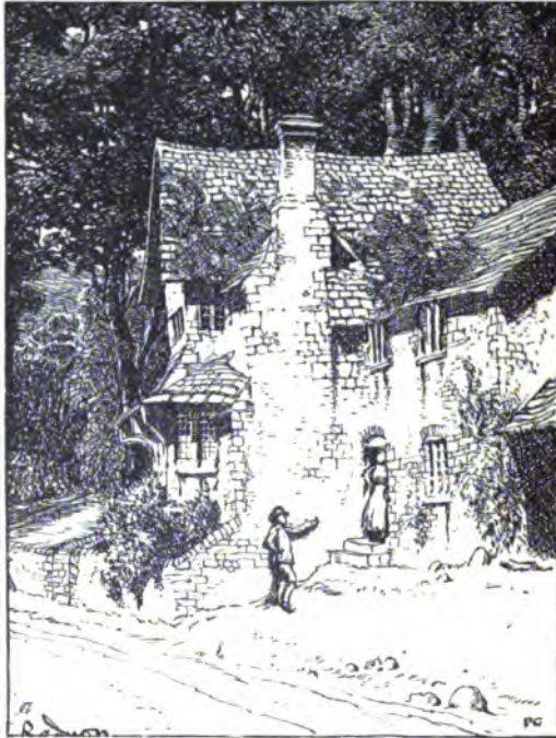
Cottage at New Radnor.
